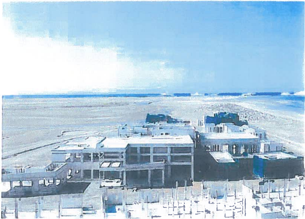
Section 1.1.1 (Ananlara Hotel): General View
