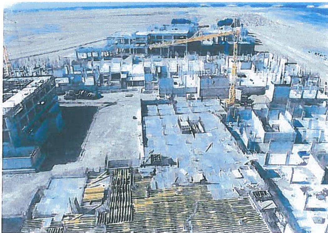
Section 1.1.2 (Amphitheatre Apartments) General View
